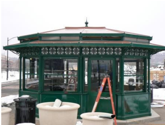
Day three of construction December 22, 2009.
