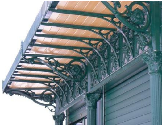
Eaveline of Kiosks with rolling shutters for windows security.
