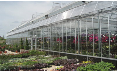
This greenhouse construction from Ludy Greenhouse Manufacturing Corp. features double roof vents for better natural ventilation, a distinct trend in garden center retailing and greenhouse growing.
